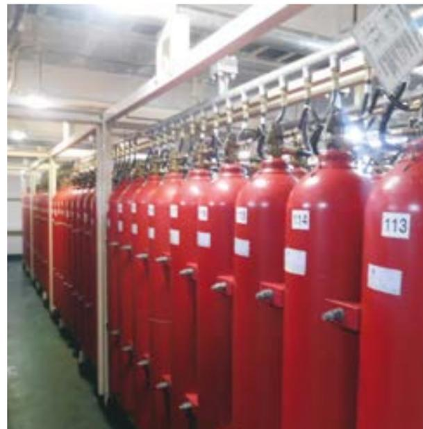
**Figure 10:** Bank of bottles for CO<sub>2</sub> fire extinguishing flooding system, source Captain Colin Fardy.
